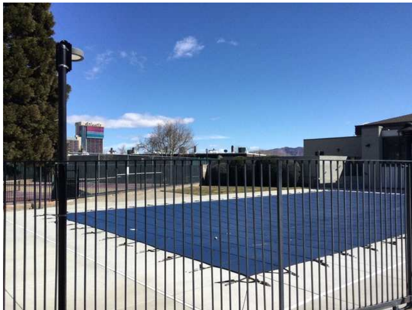
The Pool Components include Pool Re-surface, Heater, Pump, and Filter Replacement, Pool Furniture, Wrought Iron Fence Painting and Repair as needed. The Pool Restroom Remodel has also been included in the Study along with the Shade Structure Painting and Replacement. The remaining useful life of each component is an estimation only.
