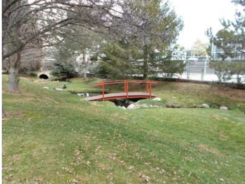
The Bridge was re-built in 2018. Future replacement has been included in the Study.
