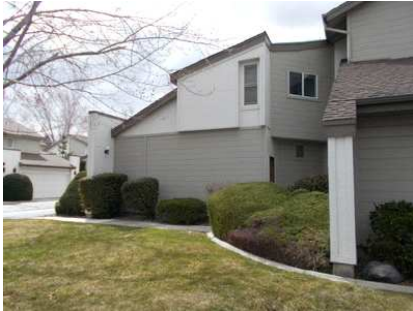
The Exterior Painting is done in phases, every 7 years, as needed.
