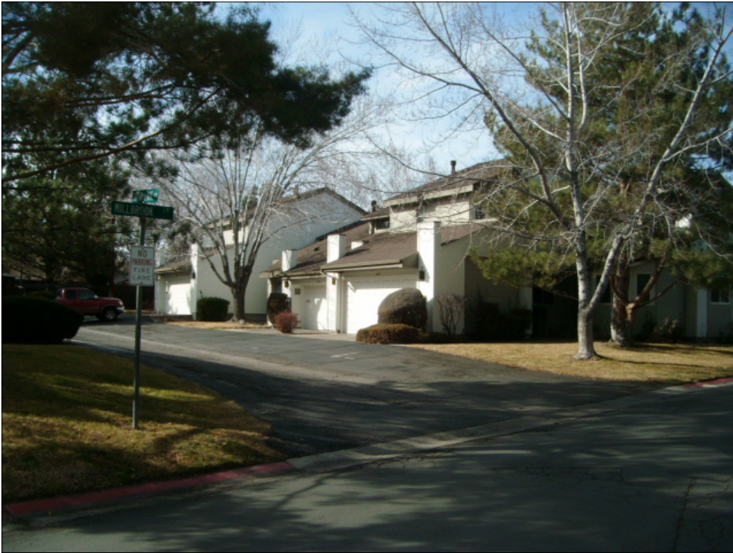
The Exterior of homes is the HOA Responsibility. A Roofing and Painting Schedule has been included in the Study. The Association is well maintained and in overall good condition.
