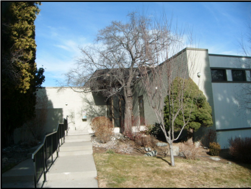
All Club House Exterior Components have been included in the Study including Painting, Roof and Windows and Door Replacement.
