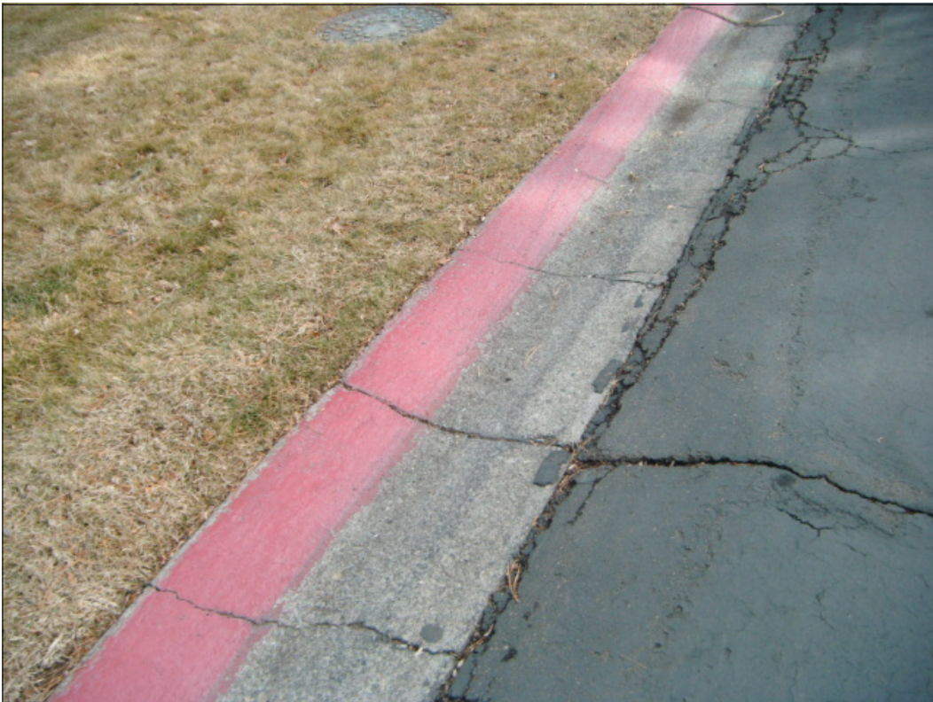
Concrete Curb/Gutters are replaced when the Roads have the overlay.
